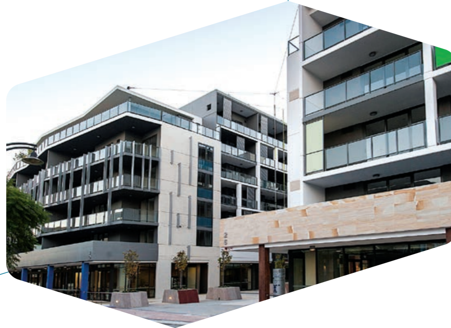
FY15 has been a strong year of project construction and completions.
