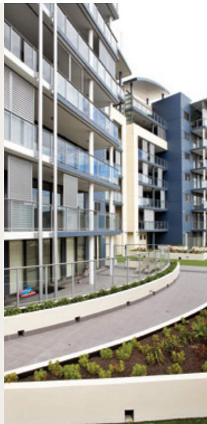
The Edge Apartments
